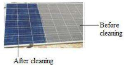
Fig.1. solar panel cleaning
