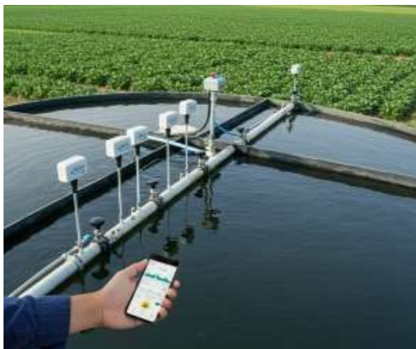
Fig. 2 Water level Monitoring System
