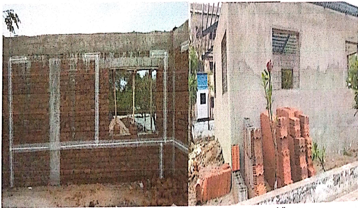
Photograph of Under Construction of "Robotic Lab"
